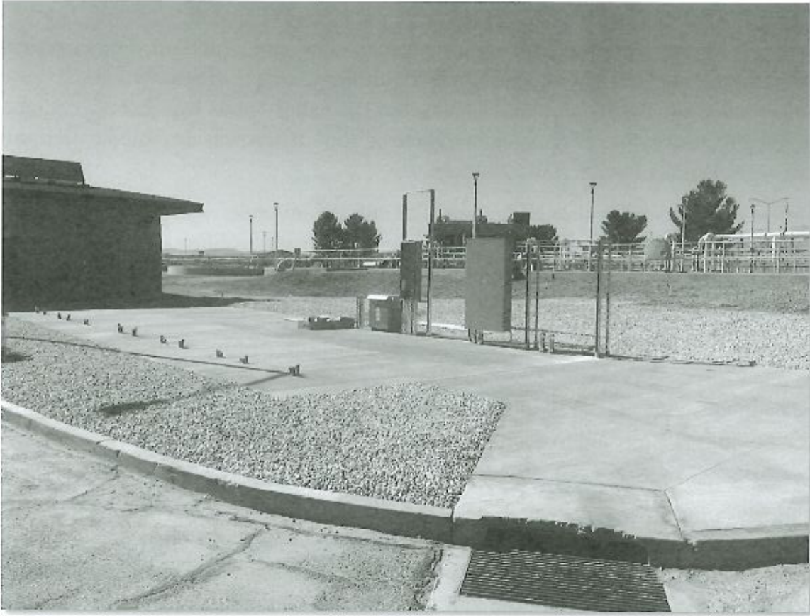
Figure 9: Prepared Flow Battery Foundation
