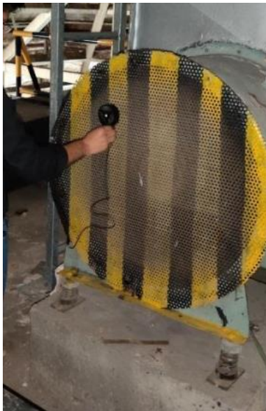
Pic no 22- Air flow measurement
