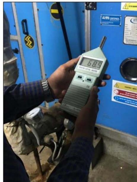
Pic no 13- Sound level measurements
