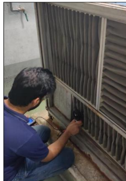
Pic 17-Air flow measurements
