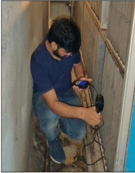
Pic no 14 Air flow measurements
