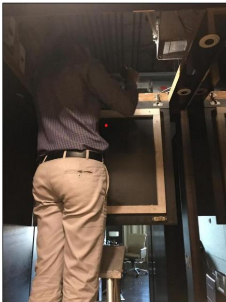
Pic 18 -Physical inspection of FCU's
